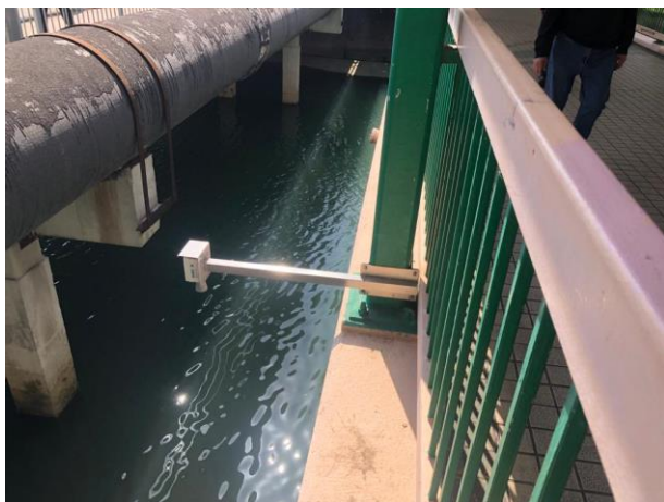
Real-time water level monitoring
